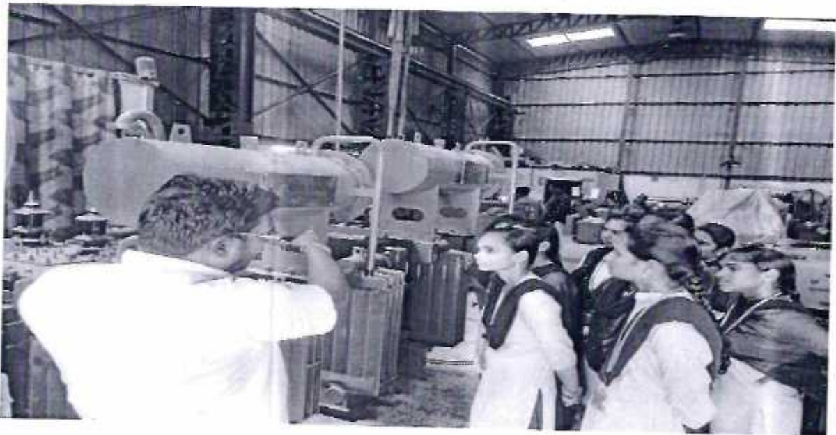
2. Explanation In the transformers
