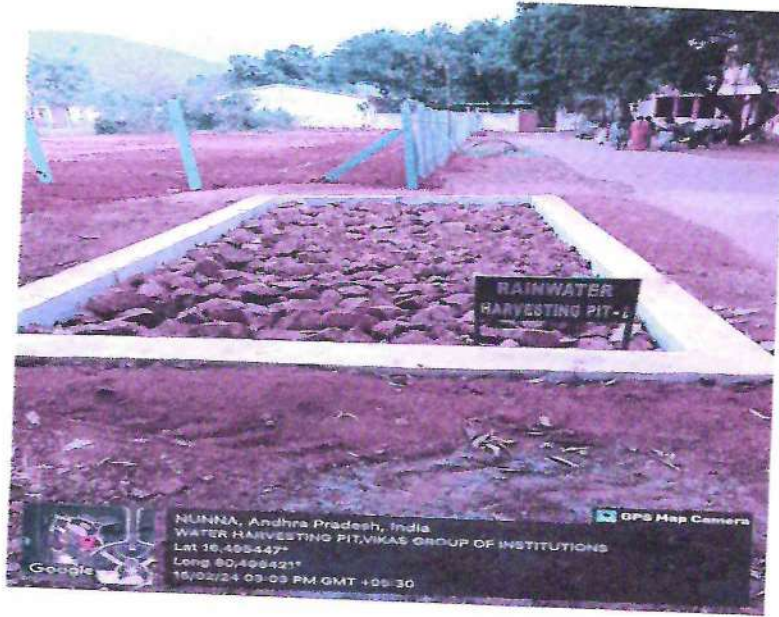
WATER CONSERVATION PITS
